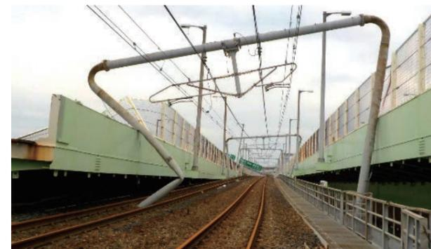
Railway damage caused by lateral shifting (about 4 m) of the outbound roadway bridge
