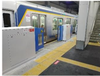
Platform gates for Nakamozu Station
