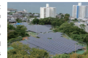
Tannowa Solar Power Plant
