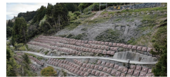
Construction to prevent landslides (within Kamikawa Station)
