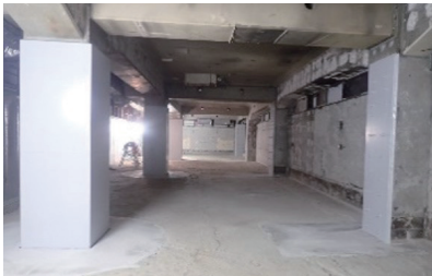
Seismic retrofitting work on the elevated bridge in Namba Station
