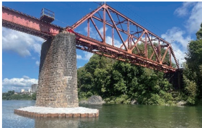
Construction to prevent scouring on the bridge pier at the Kinokawa River Bridge on the Koya Line
