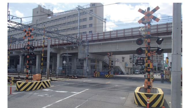
Nankai Line (in Takaishi City) continuous grade separation project construction progress
