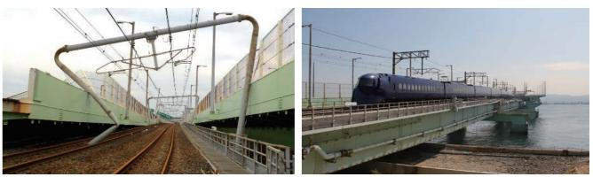
Railway damage caused by lateral shifting (about 4 m) of the outbound roadway bridge Airport connection bridge after resumption of operation
