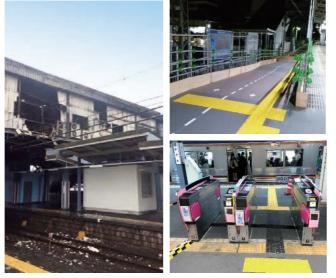
Left: Ozaki Station building after fire Right: Ozaki Station after temporary restoration with temporary passage (slope) installed above line 4 (top) and automatic wicket installed on platform (bottom)
